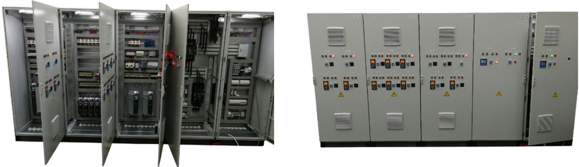
In addition to these three sections, plant is equipped with control room, which supervises all plant operations. Inside this control room, two computer stations are used for control and supervision of entire Wastewater Treatment Plant. Computer station and section control cabinets are connected in ring architecture, with optical links between control room and sections, and ethernet and siemens profibus links within each location.
