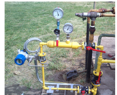
Installation of flowmeter with sandwich connection
